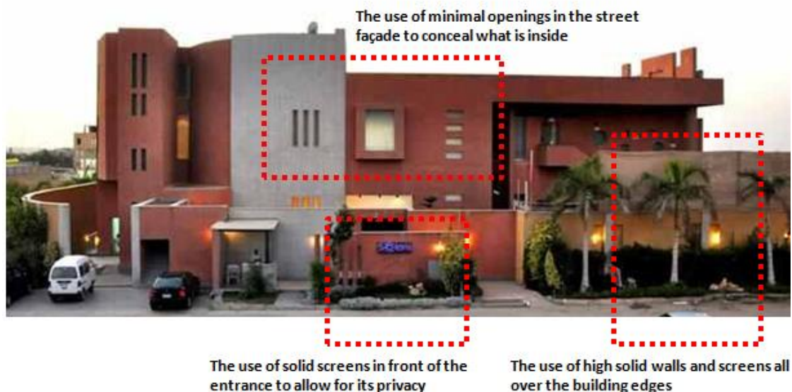
Figure 1-7: Health club entrance façade displaying how it conceals the inside facilities. Image Source: https://archnet.org/sites/6709/media_contents/73782 (assessed February 13, 2019). Image edited by researcher.
